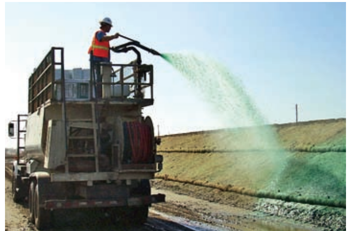
HYDROSEEDING was one of many services that Marina Landscape performed for the Bolsa Chica Lowlands Restoration Project.
